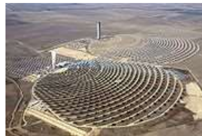
Fig. 4.4. Solar Tower Power Plants PS10 with capacity of 11MW (in the left) and PS20 with capacity of 20MW (in the right).
