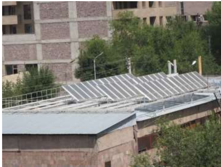
Fig. 6.11. Solar water heating system integrated with boiler house. Total area of collectors is 70 m 2 (2008)
