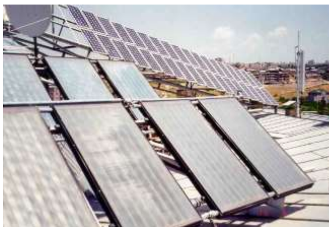
Fig. 6.7. Solar photovoltaic station and solar water heaters installed on the roof of AUA
