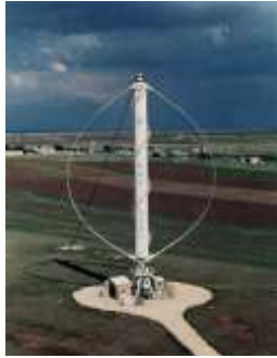
Fig. 8.3. Vertical axis wind turbine
