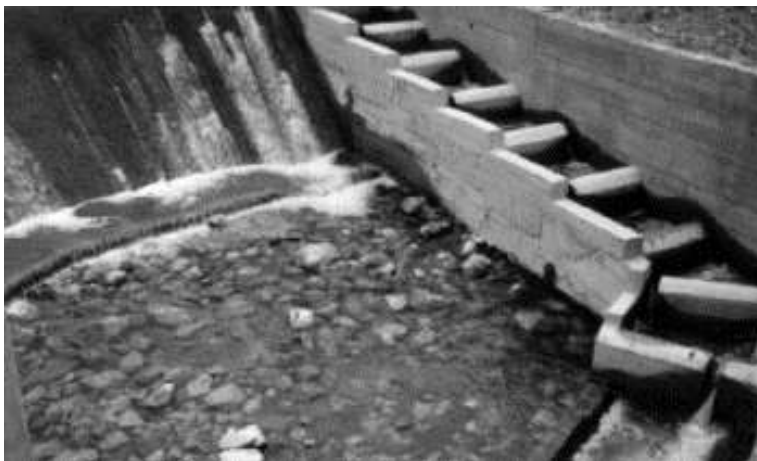
Fig. 10.12 Fishpass with vertical slots [52]
