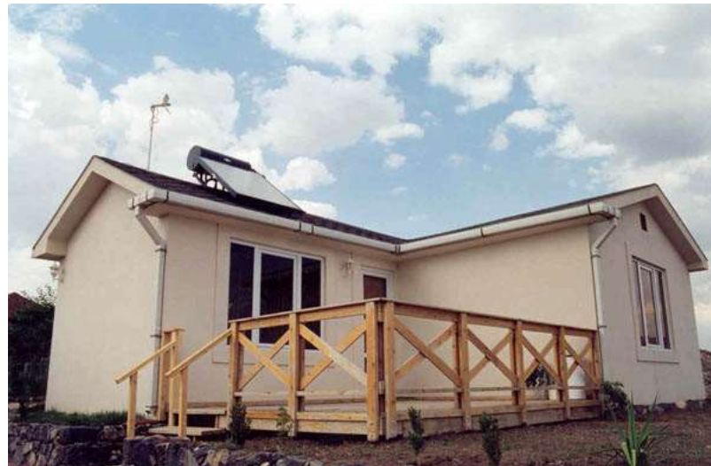
Fig. 6.5. Solar collectors installed in v. Vahagni, near Yerevan
