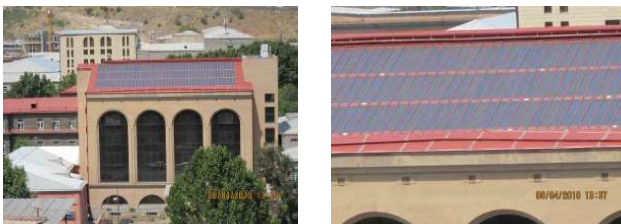
Fig. 6.9. 10 kW solar photovoltaic station installed at Armenian-American Health Center
