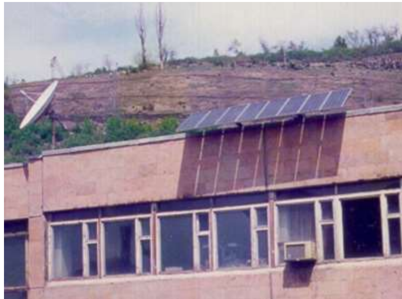
Solar photovoltaic panels at the roof of SEUA
