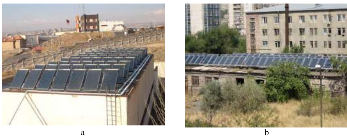
Fig. 6.10. Solar water heaters: a. Solar water heaters at the roof of Red Cross Rehabilitation Center (Yerevan); b. Solar water heaters at Narcologic Clinic integrated with back up gas boiler (Yerevan)
