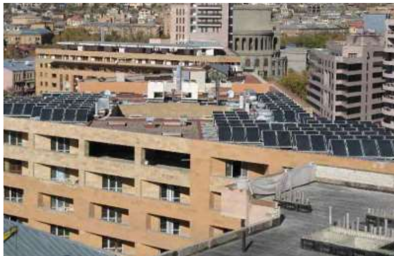
Fig. 6.6 The combined solar and water heating system at Northern ave. 10 (Yerevan)
