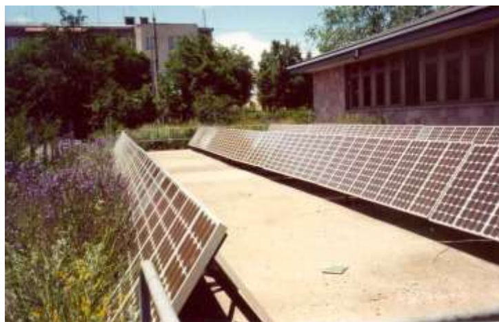
Fig. 6.4. 7.5 kW PV station in t. Gyumri
