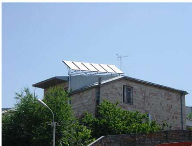
Fig. 6.12. Solar water heating system. Total area of solar collectors is 13m 2 (2006)
