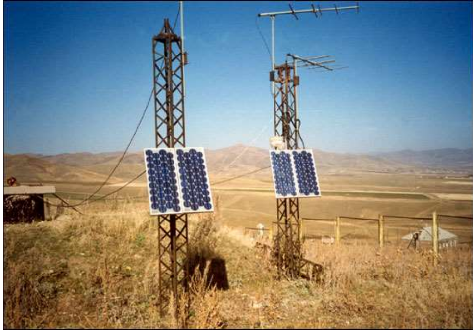
PV systems to provide seismic observation stations with electricity
