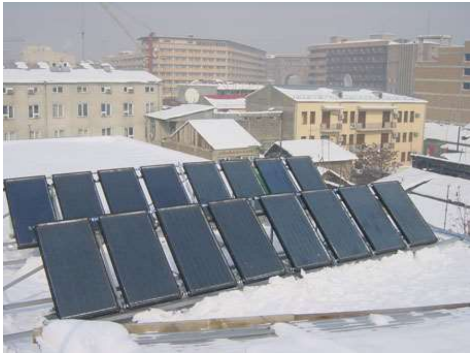
Solar water heaters at Hotel Erebuni
