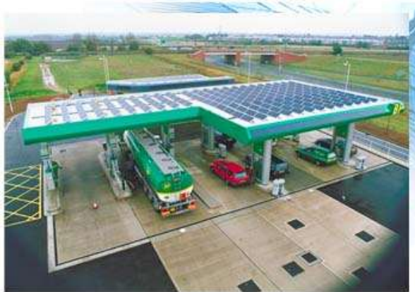
Fig. 5.9. Use of PV system at gas-filling station.
